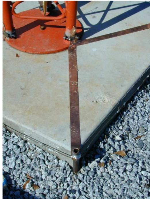
Figure 11. W8JI tower ground. Note the copper straps to pad corner ground rods and copper wire bonding the rods together. See [www.w8ji.com](http://www.w8ji.com) for this and other practical installation guidelines.
