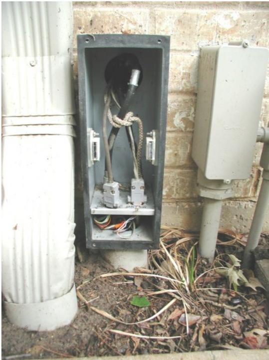
Figure 21. Feed-line entry ground. The PVC pull-box protects the connectors. The aluminum plate grounds the coax shields to the ground rod shown in Figure 10b.
