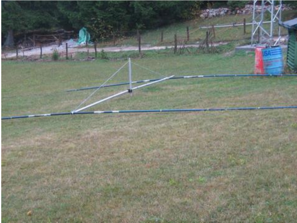
2 element 40 meter Moxon under construction
