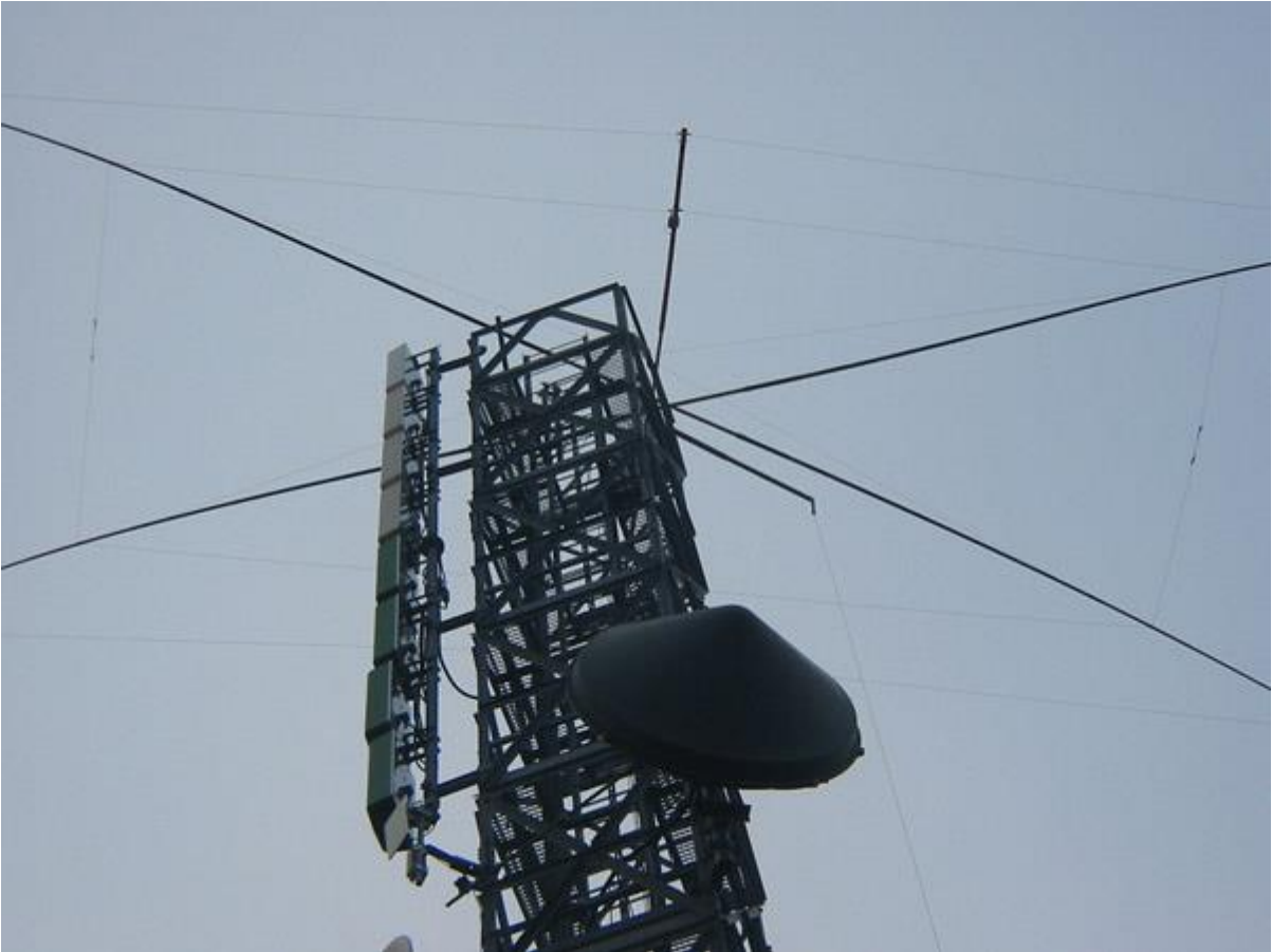
Moxon installed on the tower top. Rotor is a prosistel 3 D.
